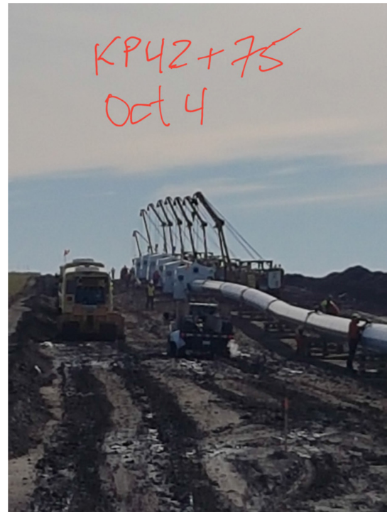
4. Welding Crew – Km 42+75 – Oct 4, 2017
