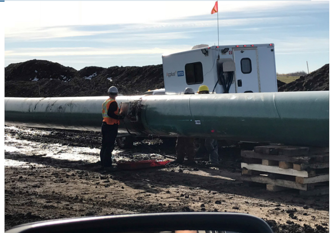
2. Welding inspectors – Km 42+750 – Oct 4, 2017
